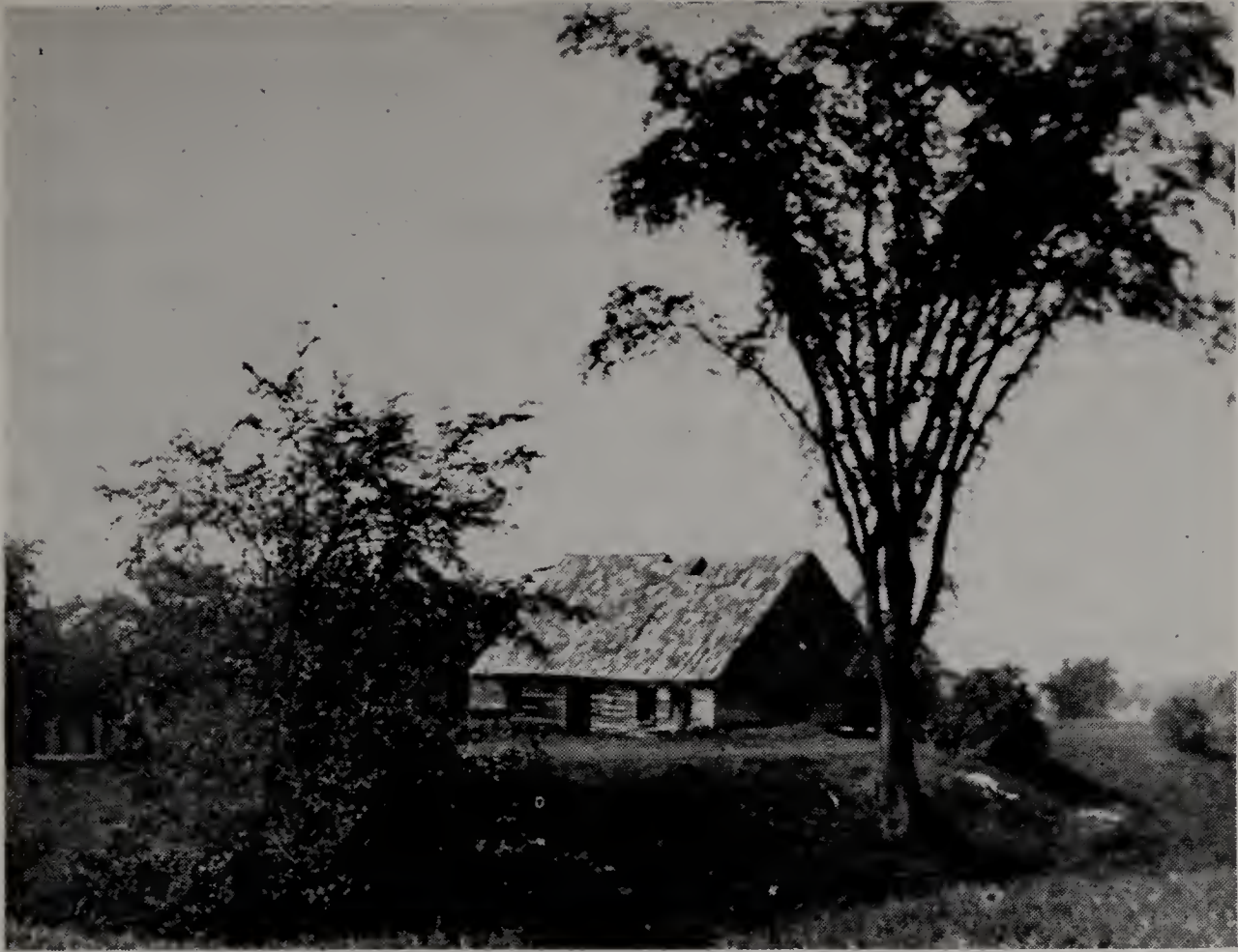
This is the home of the first settler, Col. David Hobart, on the Fairground Road, 1764 – 1900. Notice that the angle of the roof is steep, and the eaves meet the window frames.
